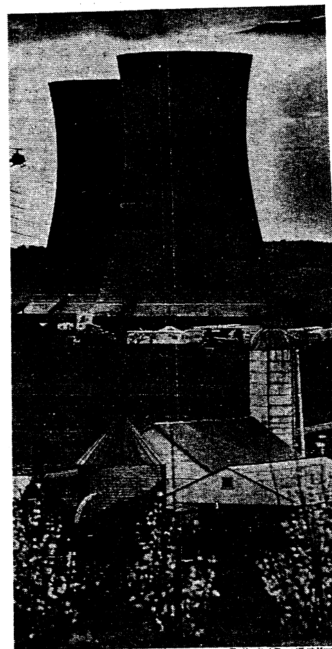
A Nuclear Regulatory Commission helicopter flew past cooling towers of the Three Mile Island nuclear plant as its crew checked radiation levels.
